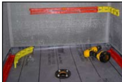
Secure StringA-Level sections to wall
