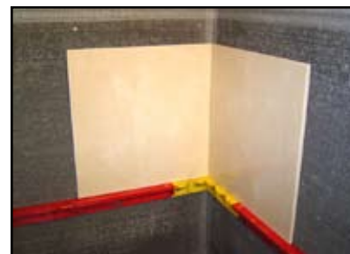
Set tile on top of StringA-Level
